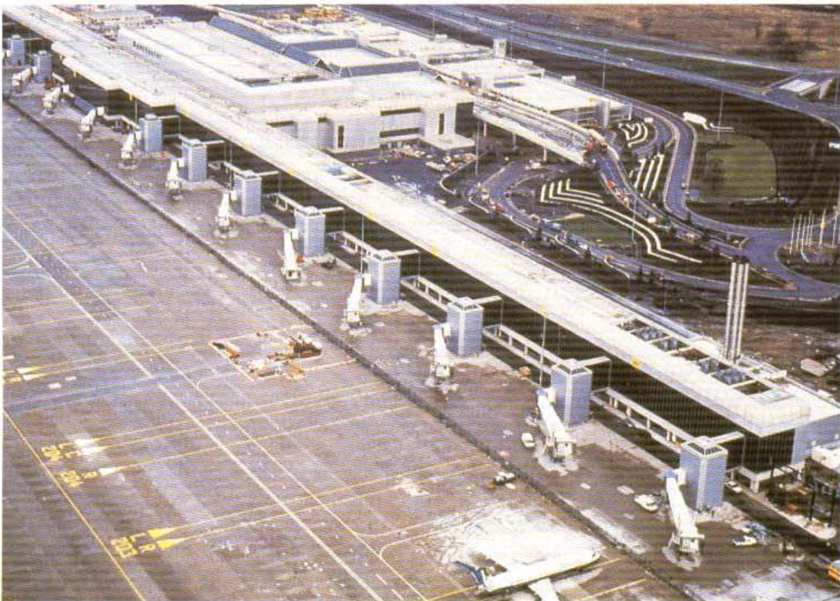
Photograph 8.3 — Manchester Airport terminal building with built-up roofing (reproduced by kind permission of D Anderson & Son Ltd)
