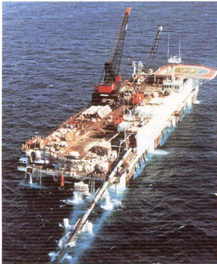
Photograph 10.7 — Marine pipeline being laid from a lay barge
