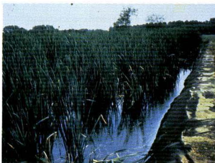
Photograph 11.6 — Geomembrane in water basin covered with 20 cm of soil to support plant growth
