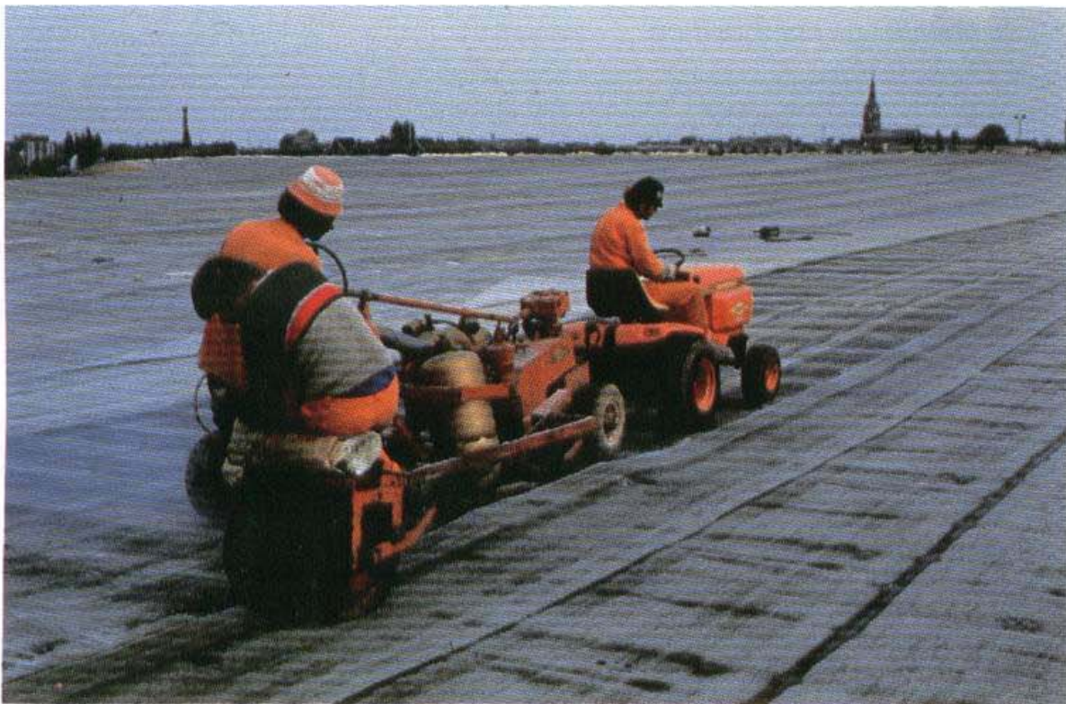
Photograph 11.5 — Heat welding of geomembrane overlaps
