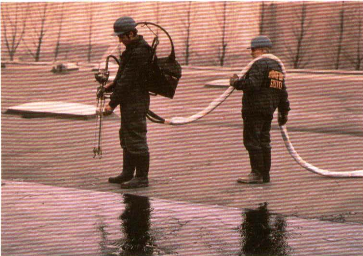
Photograph 8.6 — Spray application of the Monoform fibre/emulsion roofing system
