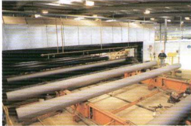
Photograph 10.3 — Priming of cleaned pipes (Photograph courtesy of British Pipe Coaters)
