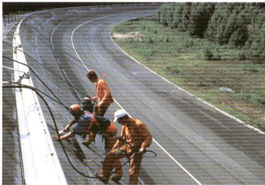
Photograph 9.3 — Application of Tixophalte on the Senlis high-speed test track in France
